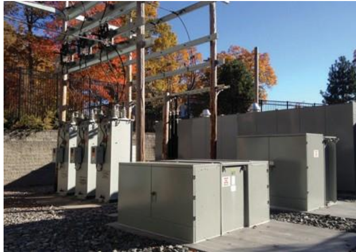
3-in-1 pad-mounted regulator with pad-mounted switchgear for bypassing to replace traditional overhead style regulators
